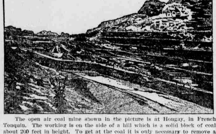
The open air coal mine shown in the picture is at Hongay, in French Tonquin. The working is on the side of a hill which is a solid block of coal about 200 feet in height. To get at the coal it is only necessary to remove a thin layer of schist on the surface. The coal is of an excellent quality, and about 1,000 tons are mined per day. This mine is conducted by a company of European capitalists, who employ 3,500 natives.
